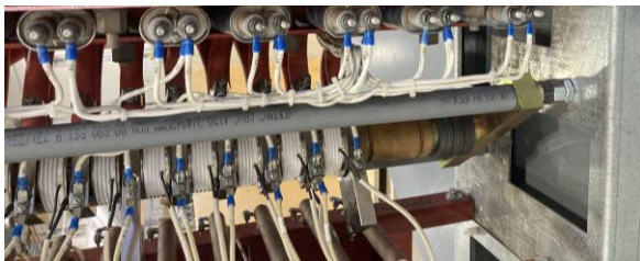
Power stack inspection / refurb
